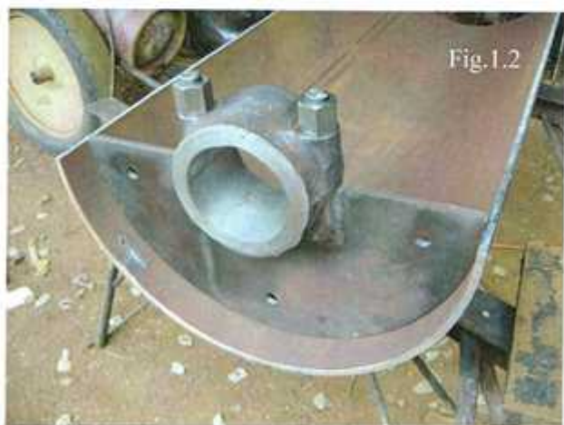
Preparing to weld the webs and main bearing housings to the upper crankcase which was made from a piece of gas pipe cut lengthwise into two identical halves.
