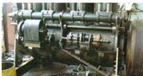
Oil pumps in place outside the crankcase.
