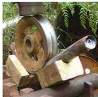
Curved outlet pipes filled with lead being bent.
