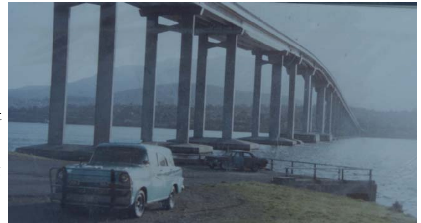
Below: The FB and the Tasman bridge after it had been repaired. That's a long way down out in the middle!
